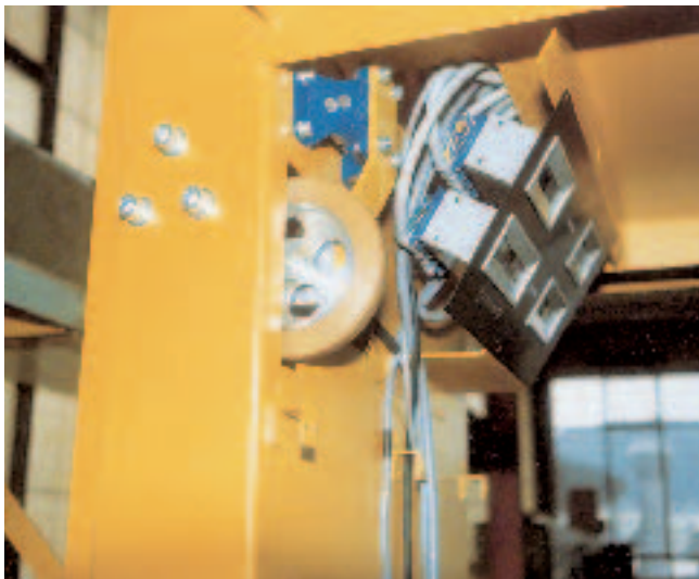
Elastic suspension of caliper roll in elevator
